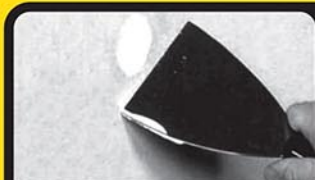
PINHOLES & HAIRLINE CRACKS
